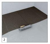
Apply wedi thin-bed mortar onto prepared surface, using 4 mm or 6 mm groove.
