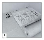
Lay out wedi Subliner Dry and cut by using a carpet cutter or scissors.
