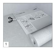
Lay out wedi Subliner Flex and cut by using carpet cutter or scissors.
