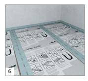
Apply wedi sealing tape and cement sealants (for outside) to corner joints and floor connections to ensure sealing. Centrally apply sealing tape onto joint.
