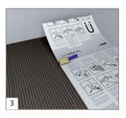
Place wedi Subliner Dry – with the printed side facing upwards – and press by using a rubber roller or wooden board.
