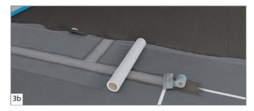
If the area is to be sealed, the board joints should be covered with masking tape. Then, apply wedi Tools sealing tape as well as adhesive to the joints, and then again apply adhesive to the whole area. Then, apply self-adhesive wedi Tools reinforcement tape 600 mm over the entire surface area..
