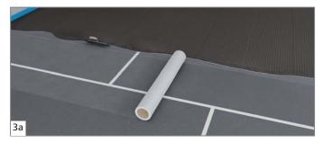
Apply the tile adhesive over the whole surface as a bonding layer. Lay the wedi Tools reinforcement tape into the tile adhesive with an overlap of 5-6 cm and bed it in with the trowel. It can then be tiled.
