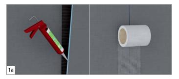
In wet areas, apply wedi 610 adhesive sealant to the joints. Then, the joints should be reinforced by using wedi Tools self-adhesive reinforcement tape.
