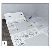
Place wedi Subliner Flex edge to edge – with the printed face upwards – and press by using a rubber roller or wooden board.
