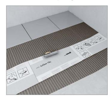
Subliner Flex serves for safe decoupling and reducing tension between top layers of ceramic tiles, slabs, and natural stone and the substrate for interior applications only. It has excellent crackbridging properties and is ideally suited for use in renovations and restorations due to its low thickness.
