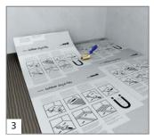
Place wedi Subliner Dry & Flex edge to edge – with the printed side facing upwards – and press by using a rubber roller or wooden board.
