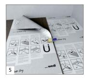
Install second membrane and press overlapping area by using trowel or rubber roller.
